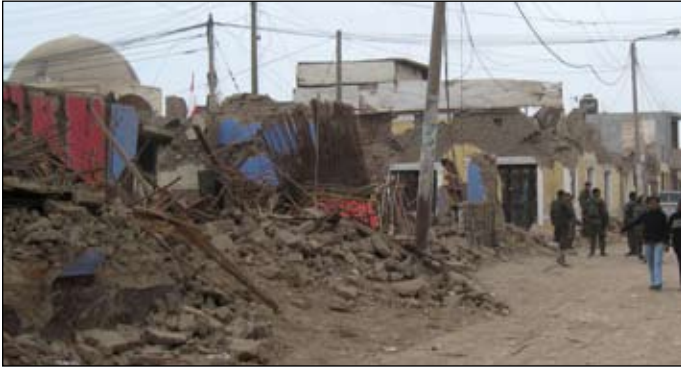
Figure 9. Street in Pisco three days after the earthquake. The house at the far right, undamaged, was made of confined masonry.
