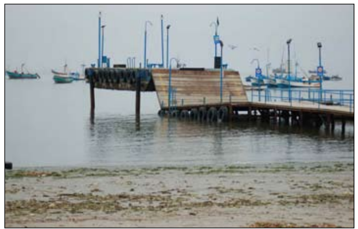
Figure 8. Paracas marina tsunami height measured based on a floating dock stuck in an uplifted position.
