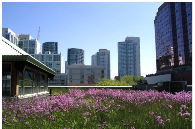
Figure 3 - Mountain Equipment Co-op, Toronto, Ontario, Canada - Inaccessible Green Roof
