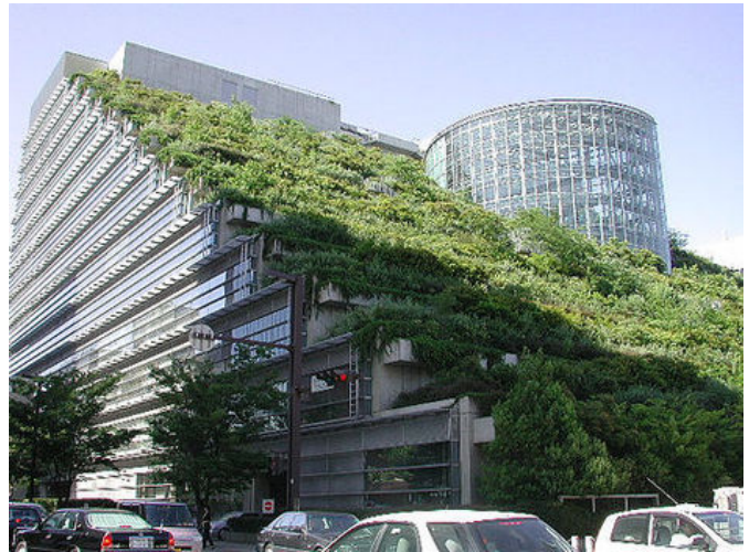
Figure 2 - ACROS Fukuoka Office Building, Japan, with Intensive Green Roof
