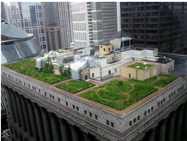
Figure 1 - Chicago City Hall Intensive and Extensive Green Roof
