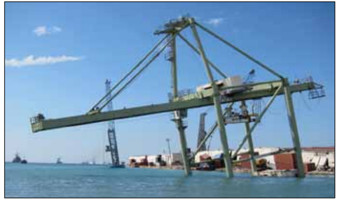
Figure 10. Submerged 15-m gauge container crane (foreground) and mobile crane (background)
