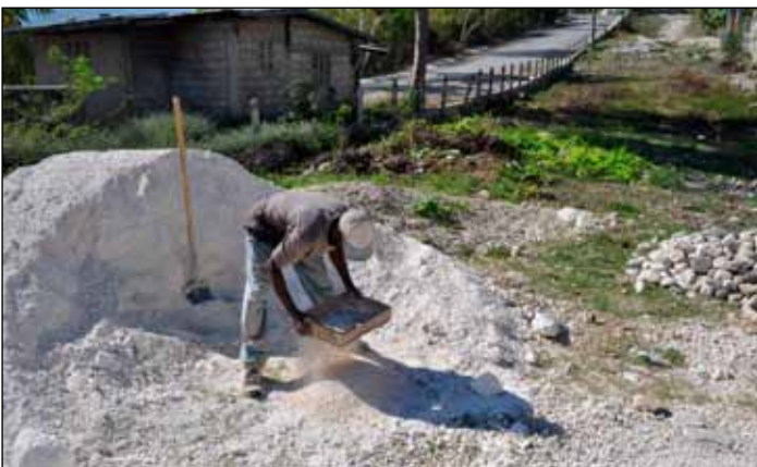
Figure 4. Hand sieving aggregate on site for mortar.
