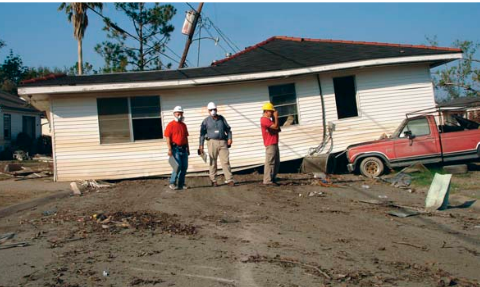
CA SAP Evaluator team assessing a house left in the street by Hurricane Katrina. Note the filter masks worn to protect the evaluators against mold.
