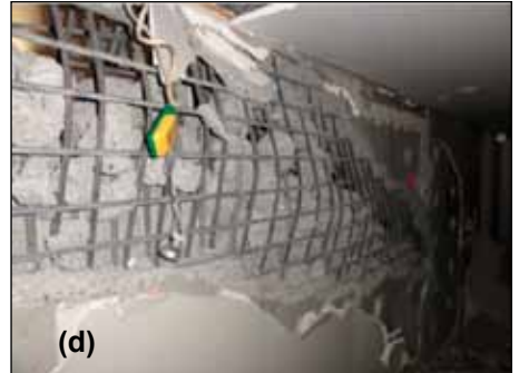
Figure 10. Examples of damage in concrete buildings: (a) column shear failure, (b) precast wall damage, (c) beam-column joint, (d) wall damage (photos: Sritharan).
