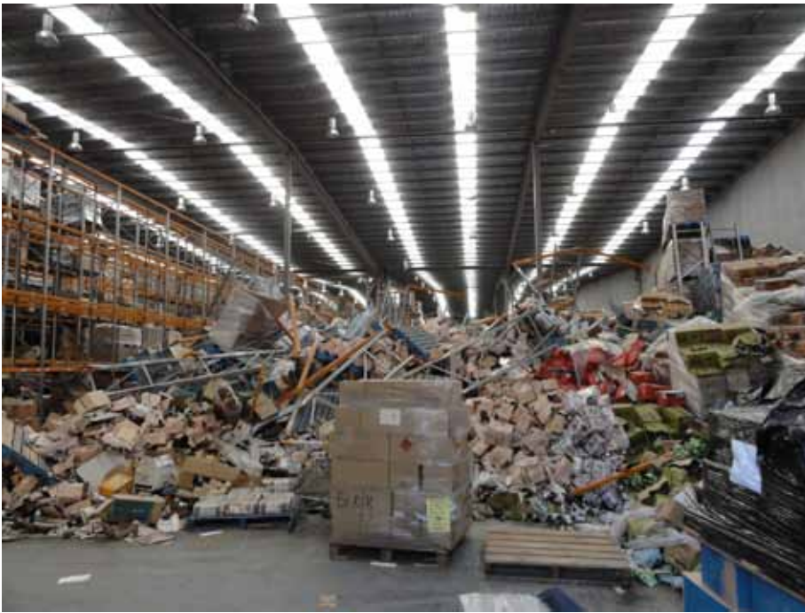
Figure 18. Collapse of storage racks (photo: Elwood).
