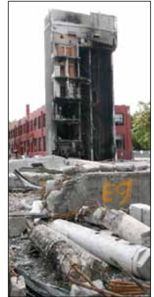
Figure 7. Collapsed reinforced concrete buildings: (a) ▲ The CTV Building and core wall (photos: Kam, Berkowitz); (b) ▼ The PGC Building (photo: Elwood).
