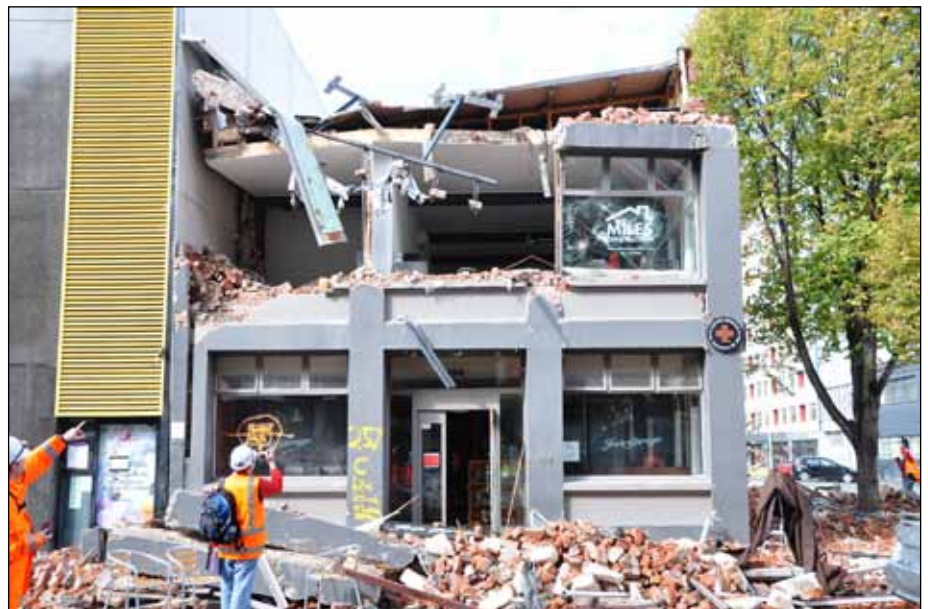
Figure 15. The EERI Team studies the performance of this heavily damaged, retrofitted URM building that pounded against the building on the left and partially collapsed (photo: Turner).
