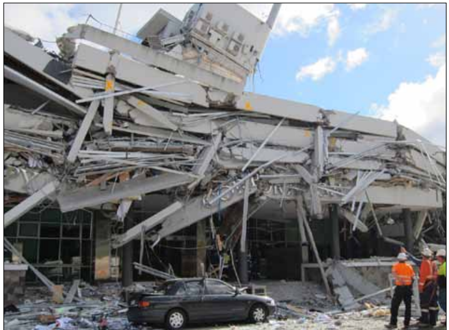
Figure 7. Collapsed reinforced concrete buildings: (a) ▲ The CTV Building and core wall (photos: Kam, Berkowitz); (b) ▼ The PGC Building (photo: Elwood).
