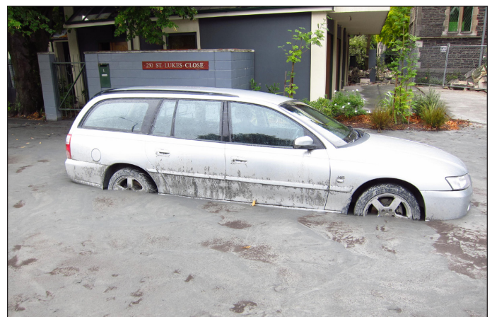
Figure 4. Severe liquefaction in the CBD (photo: Kam)
