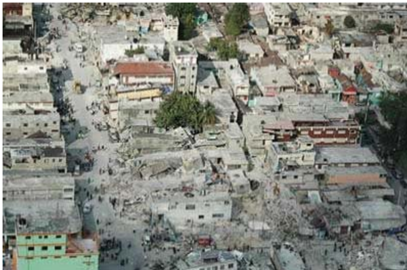
(1) An aerial photo of part of Area 8 shows the density and size of collapse. [Photos courtesy of the Los Angeles County (CA) Fire Department and USAID.]
