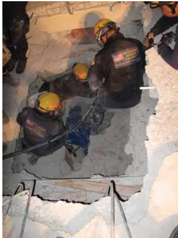
(9) Rescuers reached Makinson (under the blue tarp for protection) at the bottom of this vertical breach shaft.
