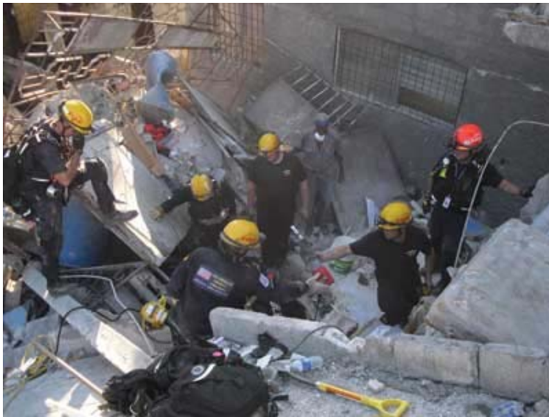
(4) USA-2 began a nine-hour rescue of three women trapped in a small survivable void space beneath a three-story collapse.
