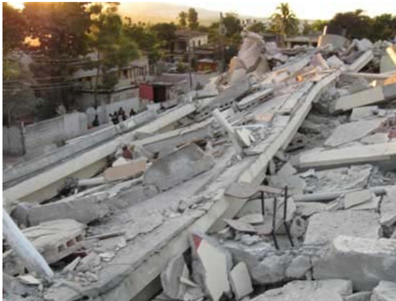
(7) Locals led a recon team to this collapsed six-story school, where a man named Makinson was trapped in a survivable void space.
